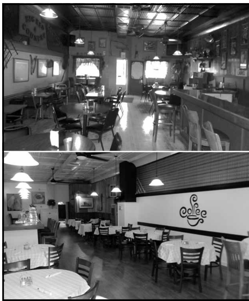
(Contributed photos) The interior of The Friendly Corner was drastically changed with both cosmetic and practical upgrades. A new commercial kitchen was installed along with several coats of paint and new flooring in the first floor of the building.
