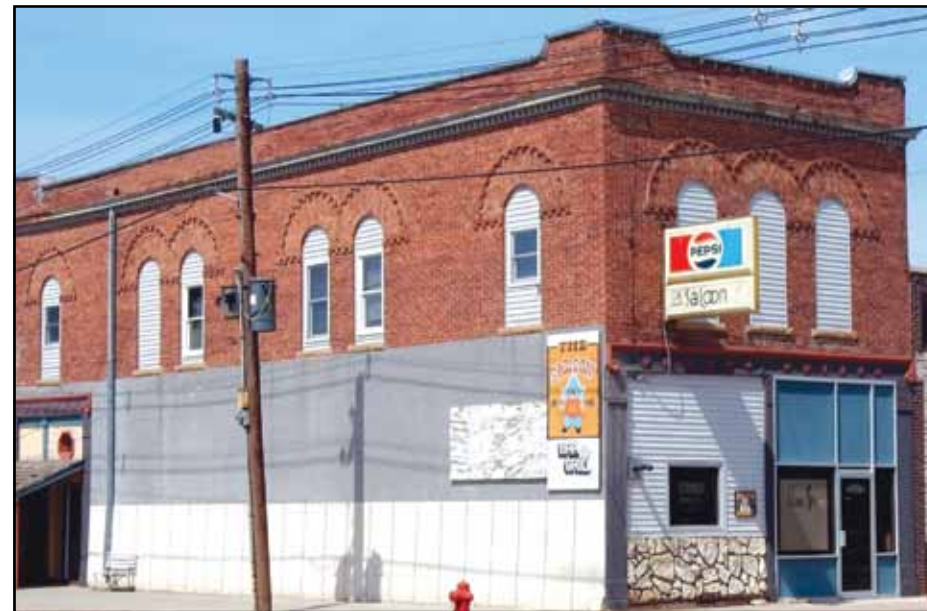
The old facade, shown here, was in need of an update that invited families to stop in and grab a bite to eat.
